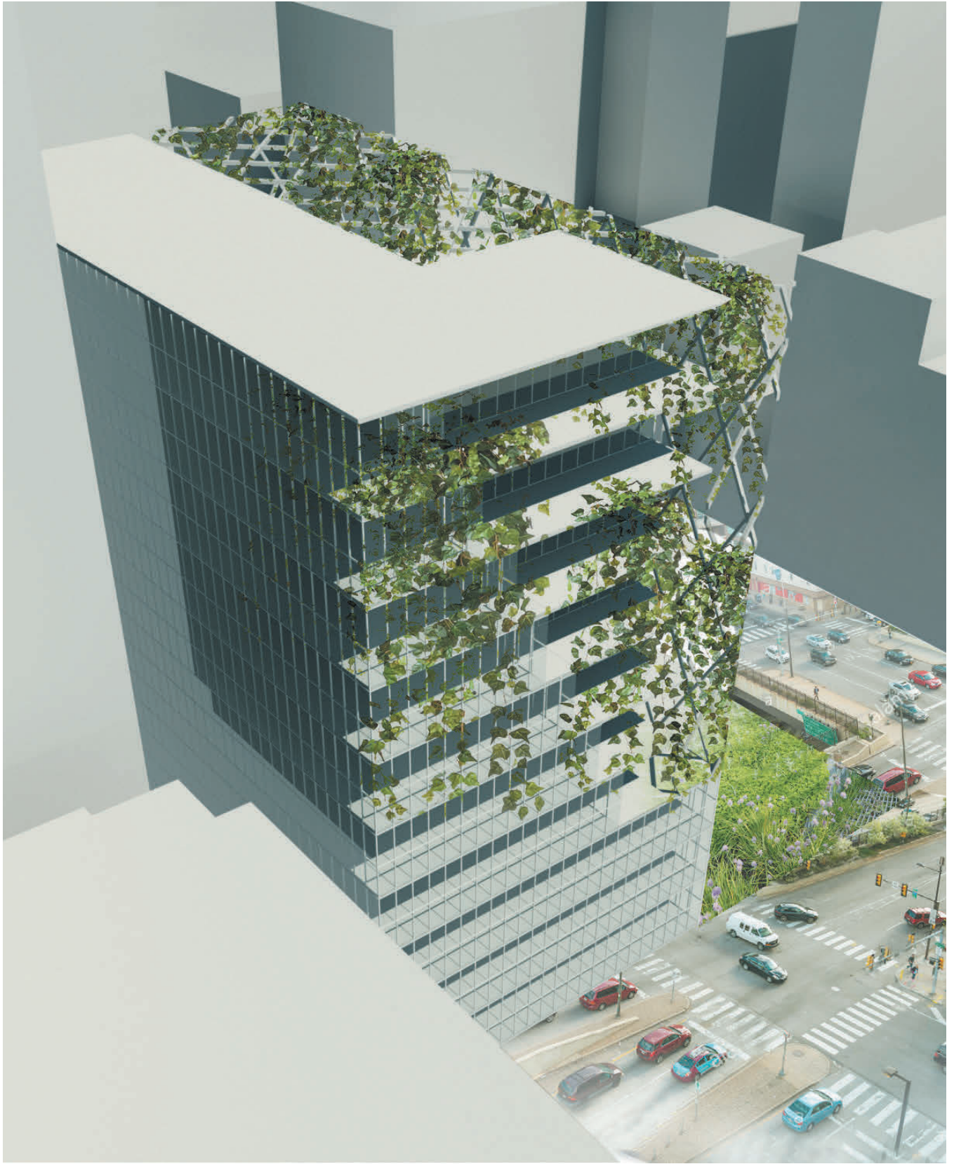
17 Eastern façade of the office building in Miami, FL, designed with deep overhangs to allow views out without compromising on its energy consumption.
